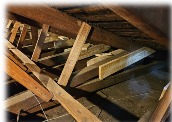
Rafters in the historic St. Paul's structure were in need of repairs before the new roof could be completed.
